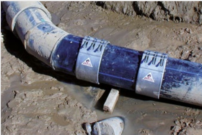
Tensile-resistant repair of a pipe section made of polyethene.
