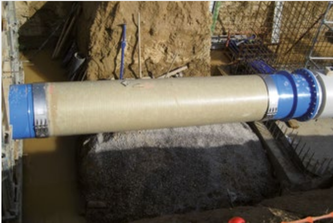
Connection of two distribution chambers with one GRP pipe section.
