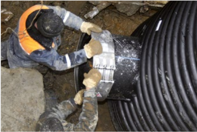
Tensile-resistant installation for an inspection chamber made of polyethene.
