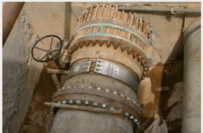
Installation of a GRP pipeline for water supply.
