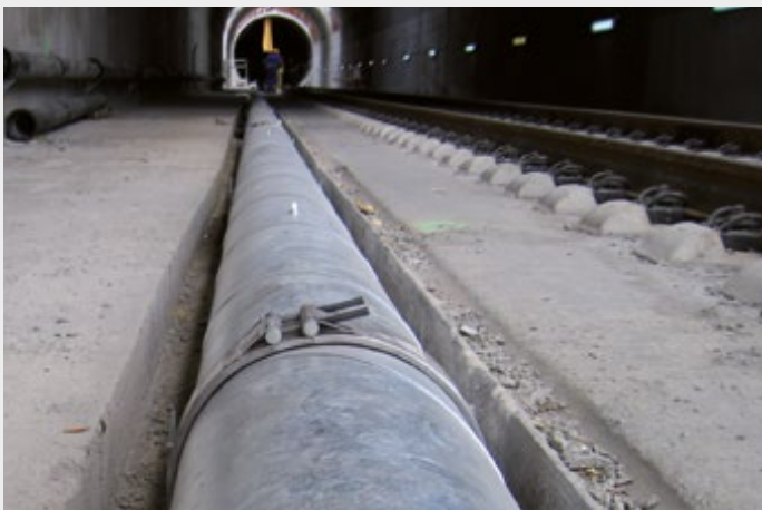
Installation of a galvanized steel pipe for air supply.
